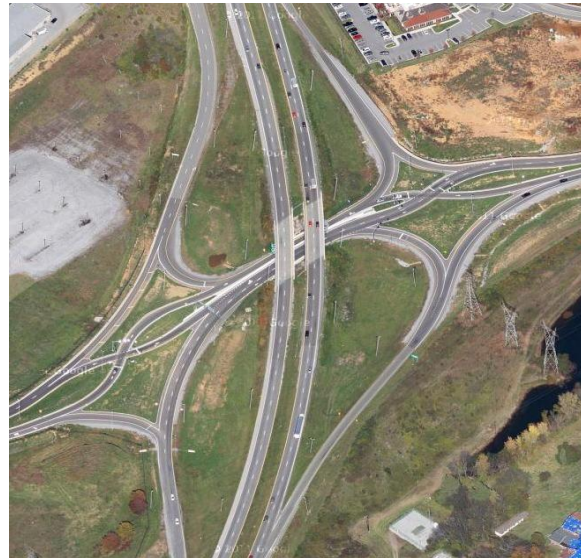
FIGURE 7(B): Bessemer St. @ US 129 Alcoa, TN
